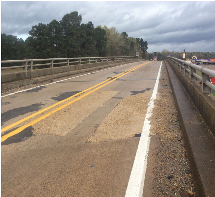
PHOTO 1 Description Deck, span 4 both lanes, with the worst being in the south bound Rt. lane.
