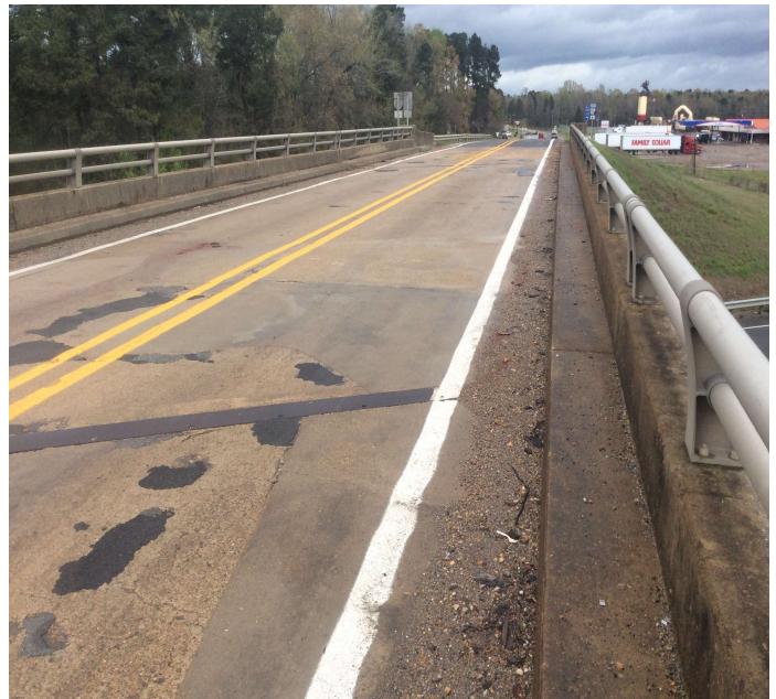
PHOTO 2 Description Deck, Spans 1 & 2, looking north against log, have numerous pot holes that are patched with cold mix both lanes.
