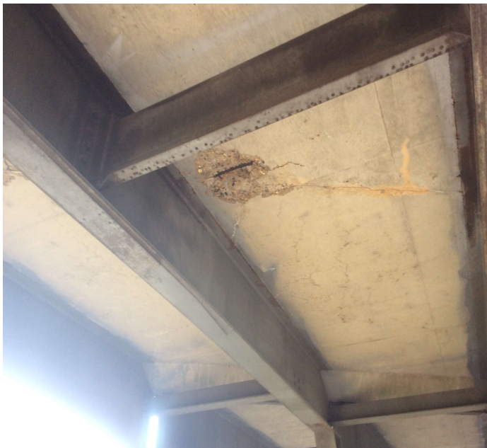
PHOTO 1 Description Spall in Soffit span 1 @ construction joint.
