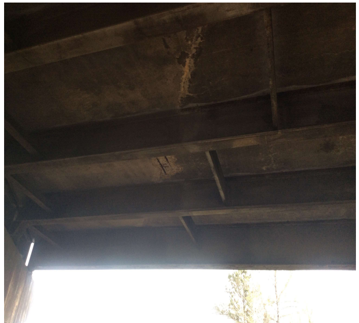
PHOTO 2 Description Spall in Soffit span 4, @ construction joint
